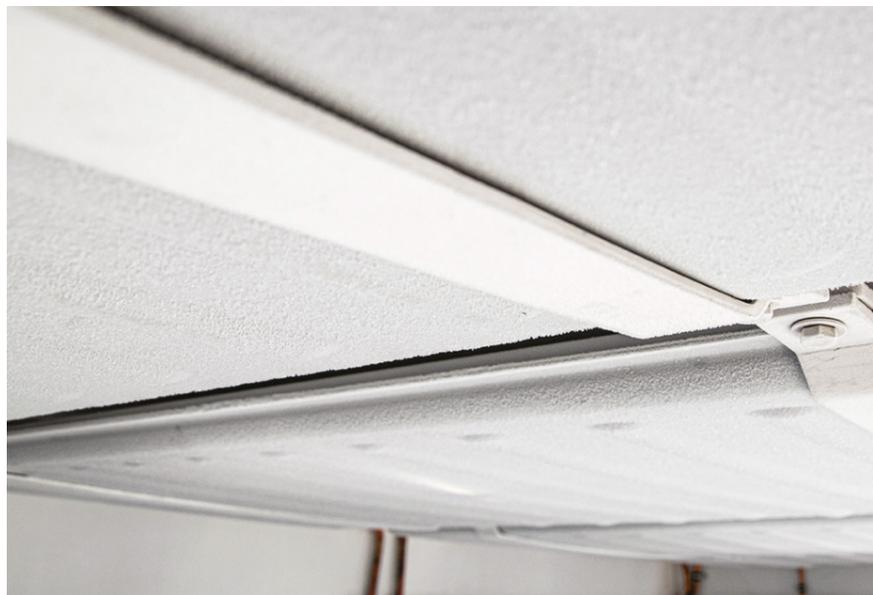
Eutectic plate sheets, which are cold pressed in specially designed molds, are welded to high standards after the internal pipe installations are laid.
